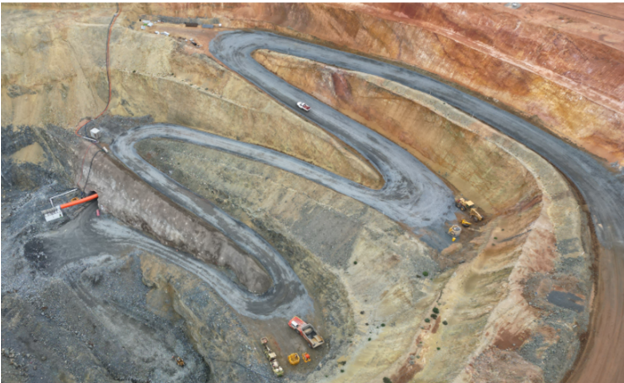
Figure 3 - View of Riverina Portal and access ramp
