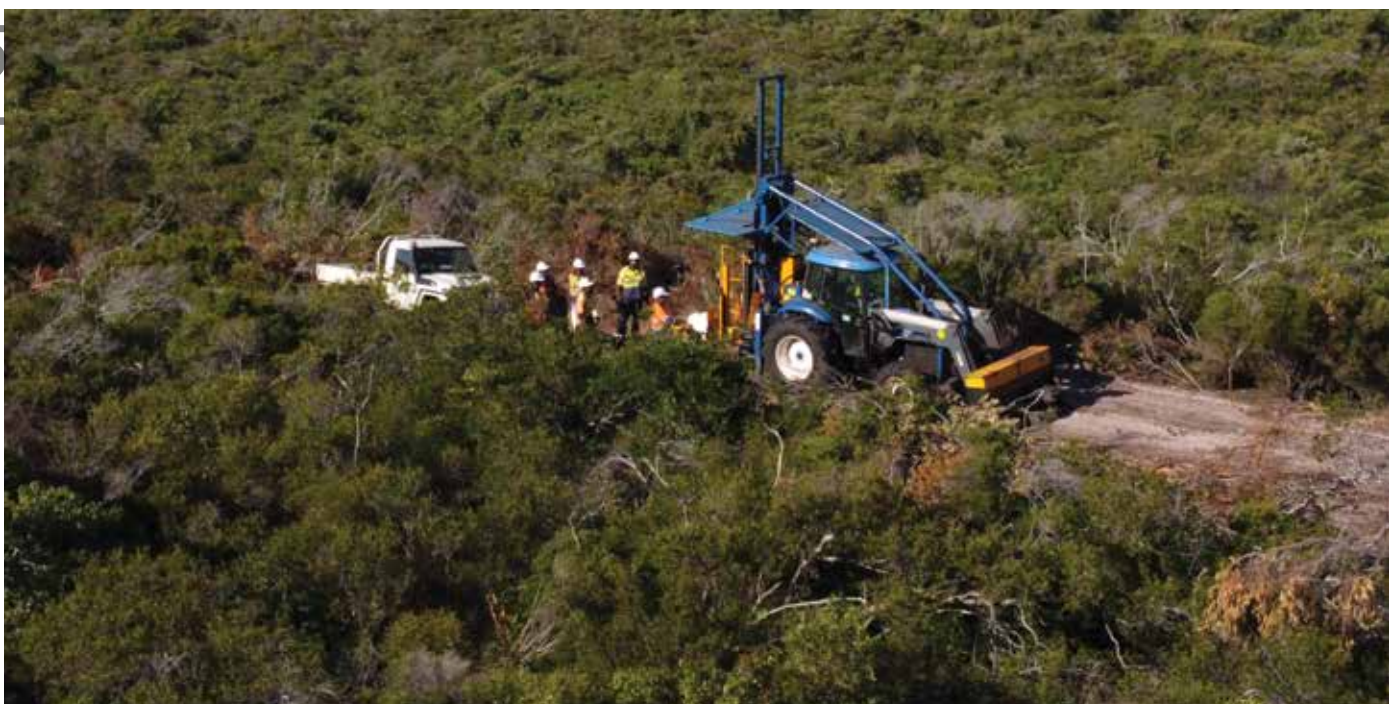
Figure 3: Tractor Mounted Vacuum Drilling rig used at Cape Flattery
