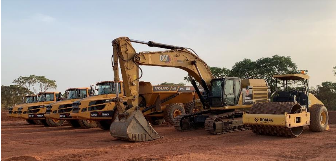
Corica's early works fleet (Volvo ADT's and Cat excavators). Long term fleet is yet to arrive and includes CAT6030s excavators coupled with CAT777 trucks
