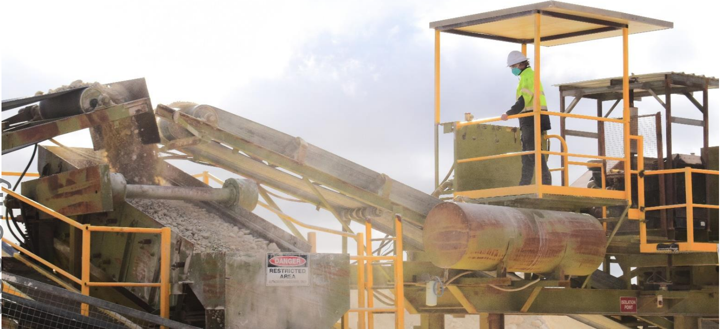
Figure 3: Classic Minerals Kat Gap crushing circuit - part.
