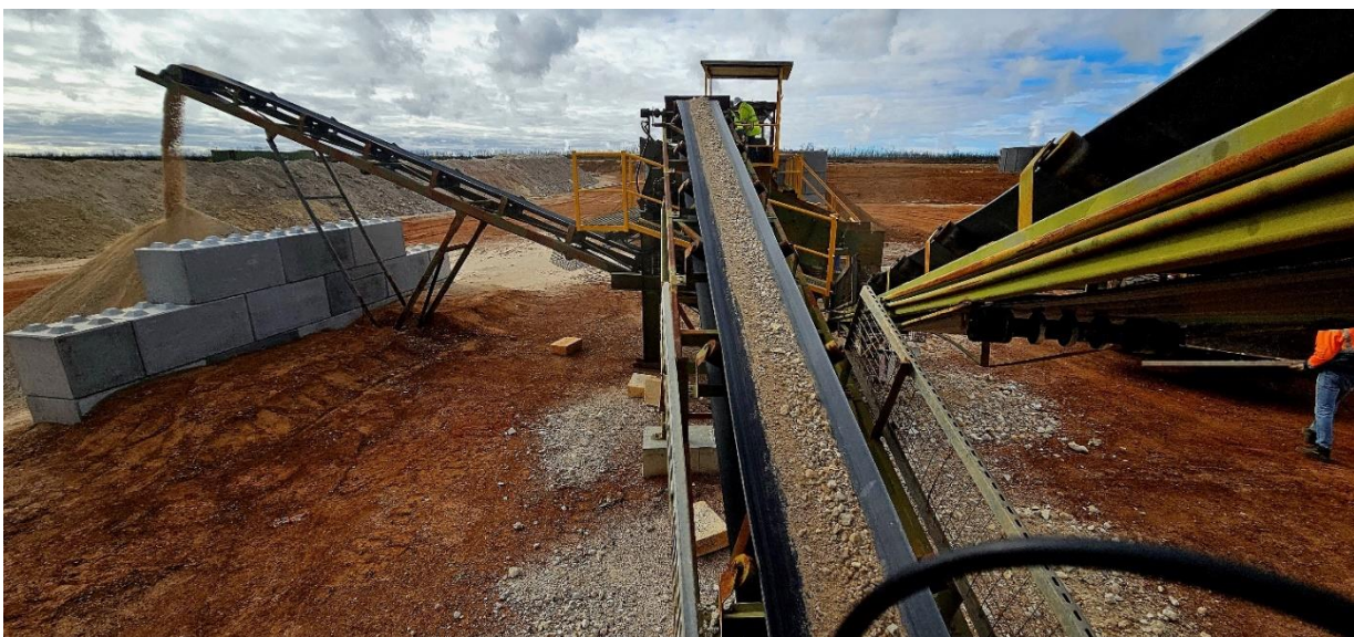
Figure 4: Classic Minerals Kat Gap crushing circuit – part.
