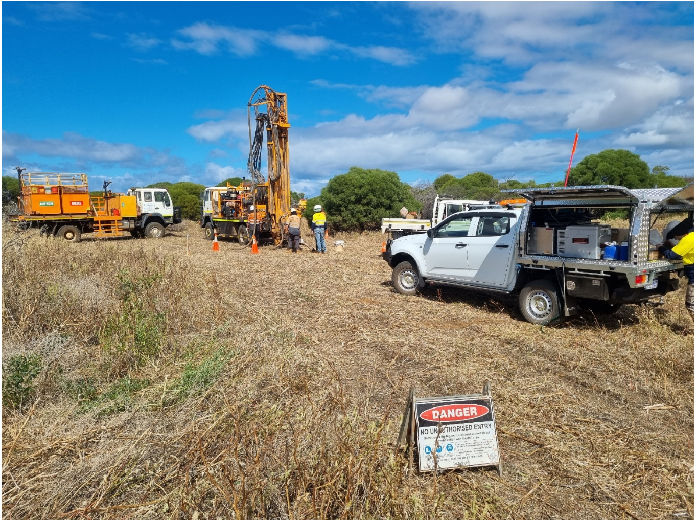
Figure 5: Bostech drilling rig on site
