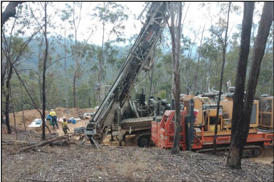
Photo 1: Geos and drilling team on site - Stage 2 RC drilling.
