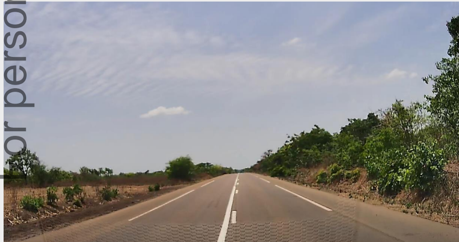
Typical road condition - Tingrela area, Côte d'Ivoire
