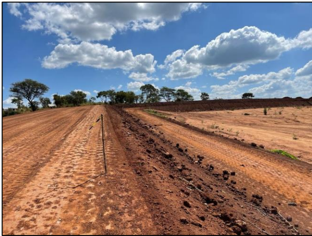
Figure 2: Completed clay-lined embankment walls (left) and in progress (right) of the pre-depositional area of the TSF in preparation of the installation of the HDPE liner.
