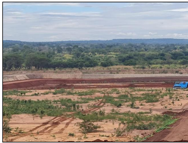
Figure 2: Completed clay-lined embankment walls (left) and in progress (right) of the pre-depositional area of the TSF in preparation of the installation of the HDPE liner.
