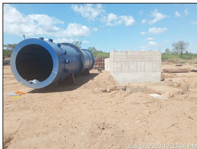
Figure 2: Drum Scrubber and attritioning mills on site (left) and two sections of the rotary drier in temporary laydown near the mounting plinths (right).
