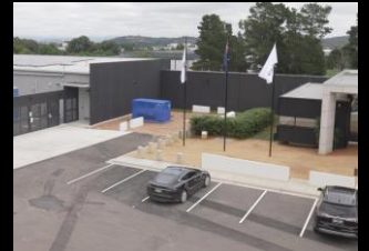
Intellicentre 5 South Bunker, Canberra
