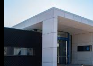
Intellicentre 4 Bunker, Canberra
