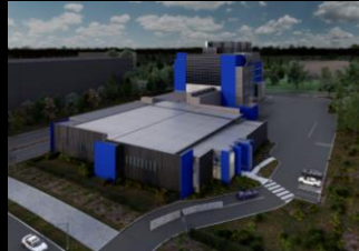
Intellicentre 3 East Macquarie Park
