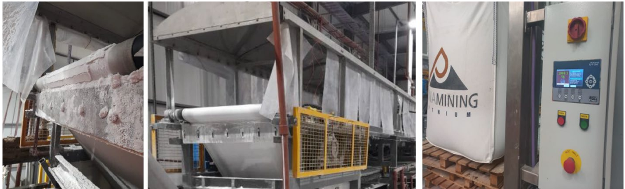
Figures 4-6. Rincon Lithium Project – 2,000tpa Operation Commissioning Works
