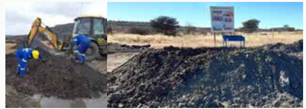
Figure 6: Tshipi's bioremediations facility project
