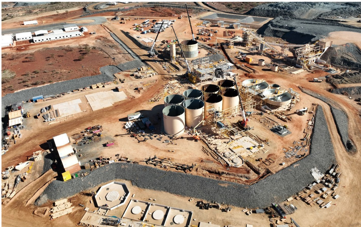
Figure 4: Processing Plant construction progress 21 May 2023.
