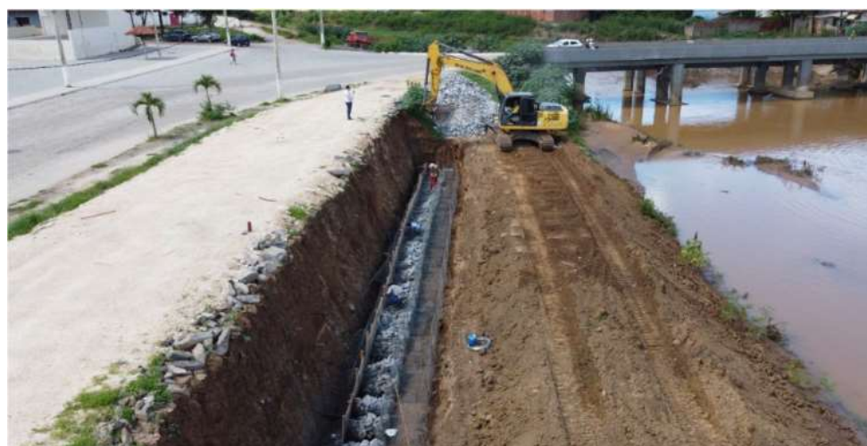
LRS funded levy wall in Salinas built December 2022
