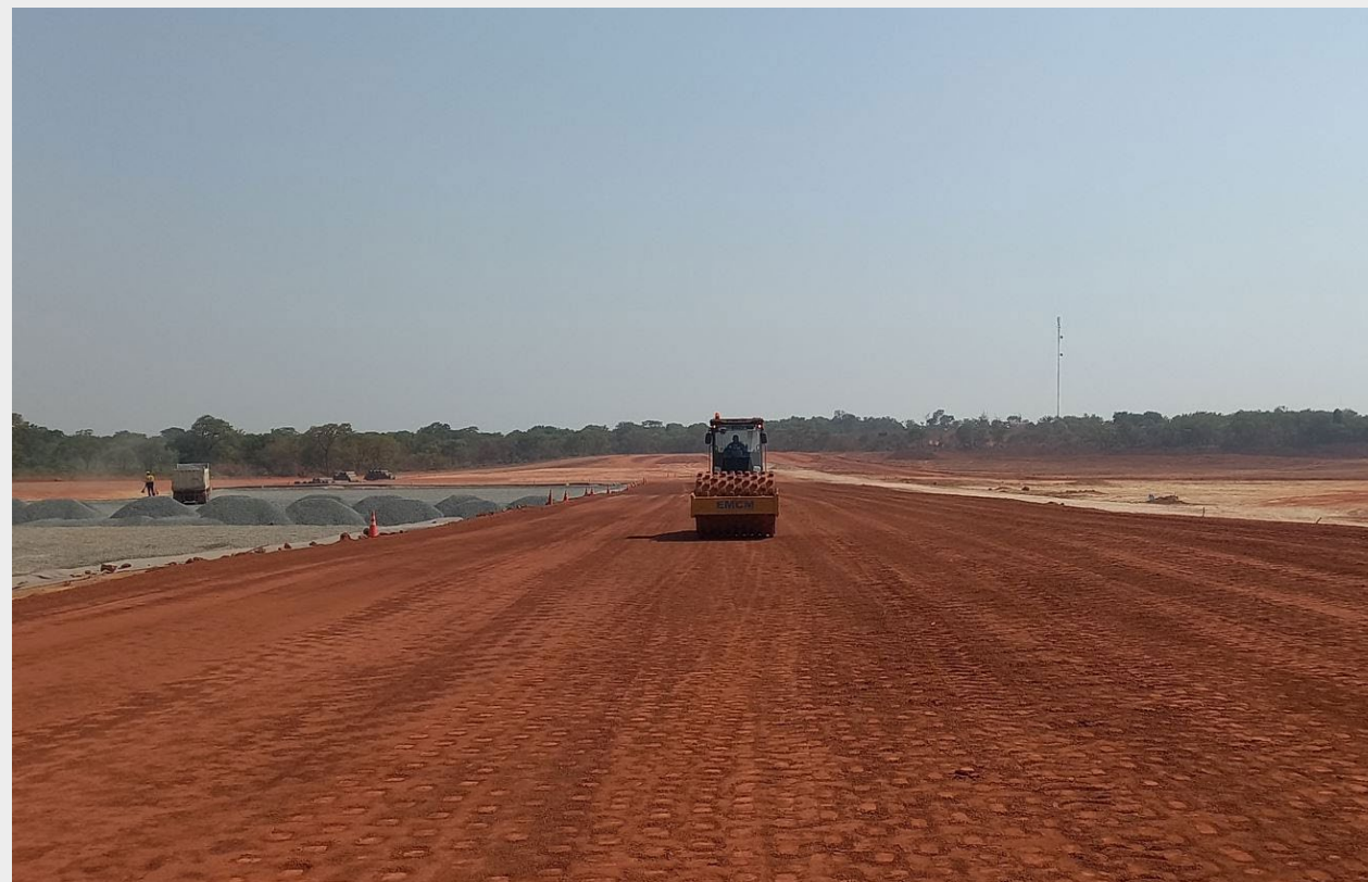
TSF wall construction with drainage layer being installed
