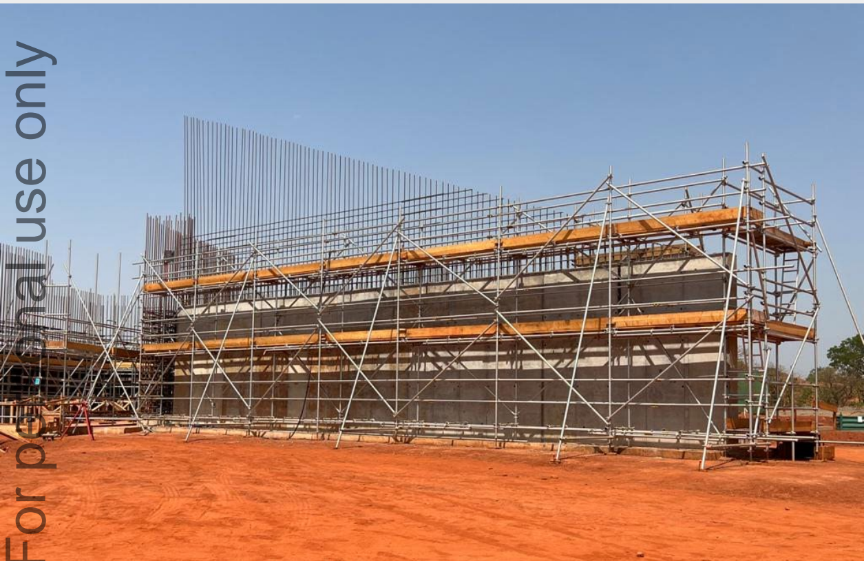
Primary crusher wall scaffolding
