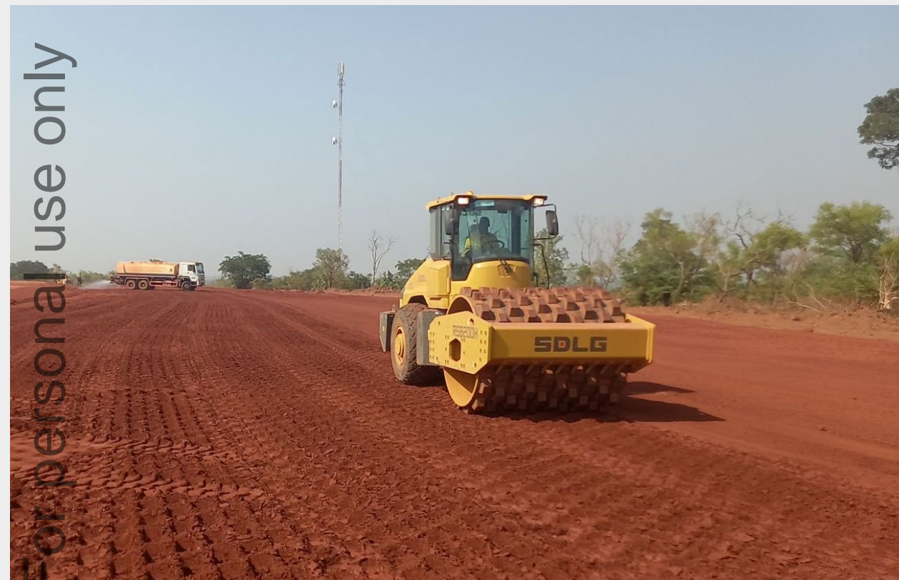
Civil earthworks in readiness for the permanent camp installation
