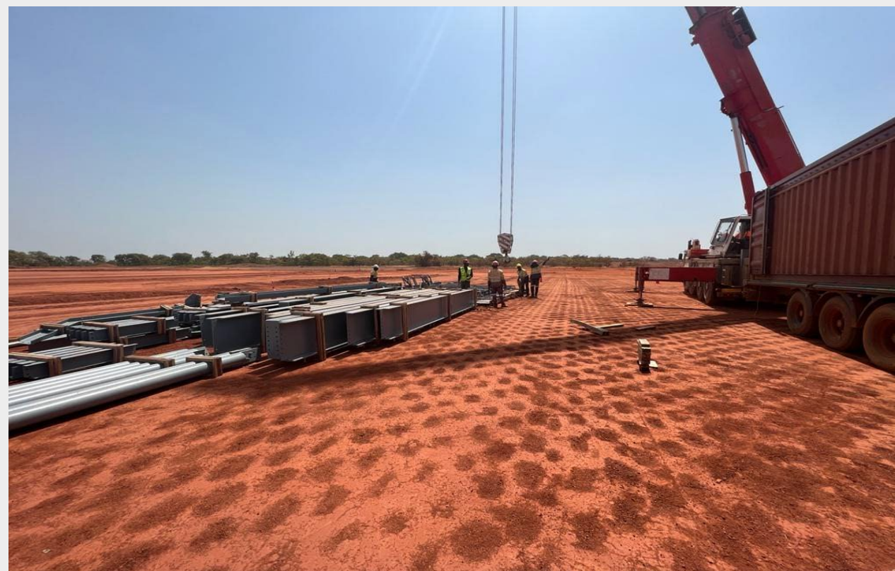
Unloading of the first steel on site
