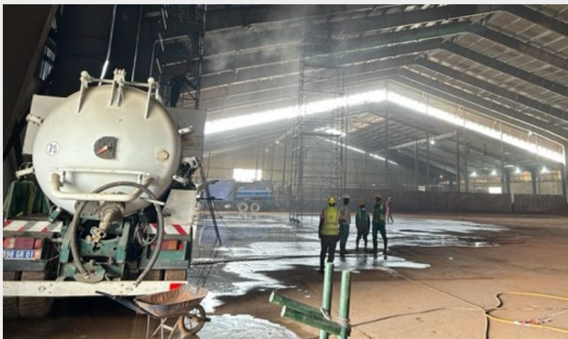
Shed cleaning in readiness for DSO
