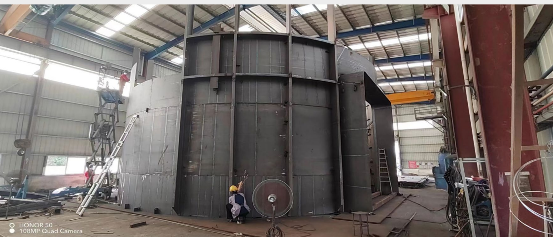
Steel plate work, Asia
