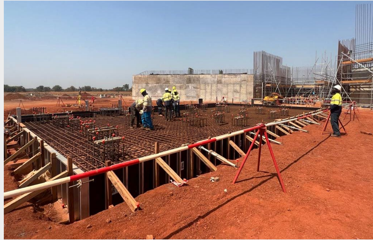
Primary crusher foundation with main chamber in background
