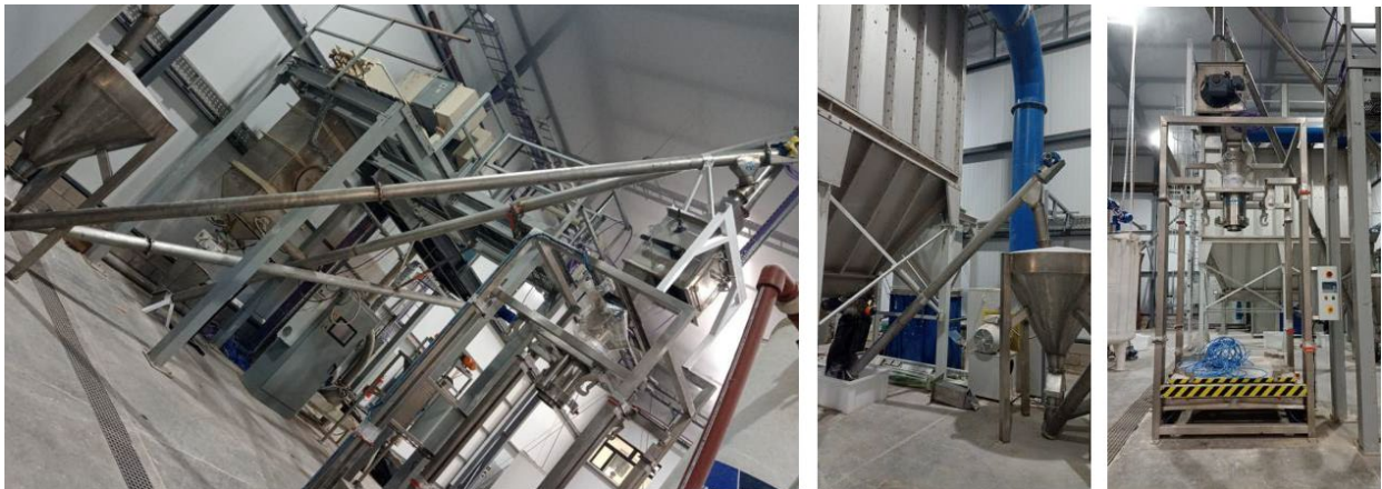
Figures 2-4. Rincon Lithium Project – 2,000tpa Operation Commissioning Works
