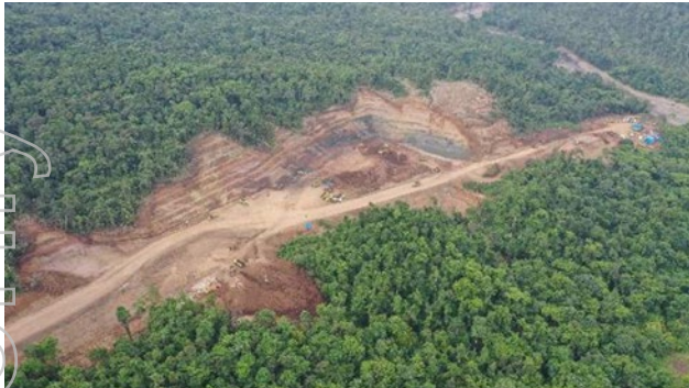
APL segments of haul road to IMIP under construction
