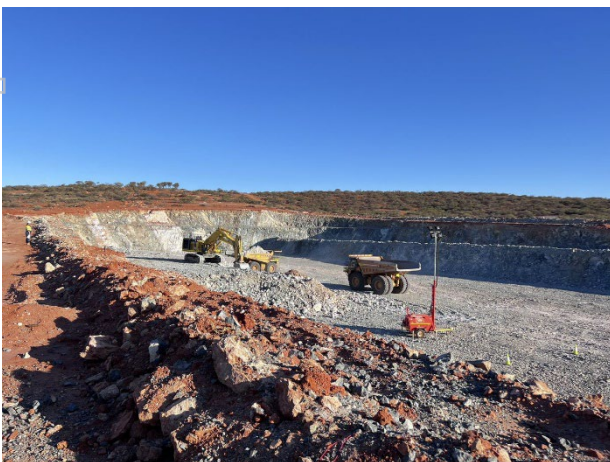
Figure 3: Formation of the Mt Mann box cut
