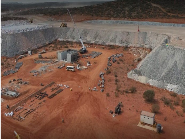
Figure 7: Run-of-Mine pad with primary crusher foundations
