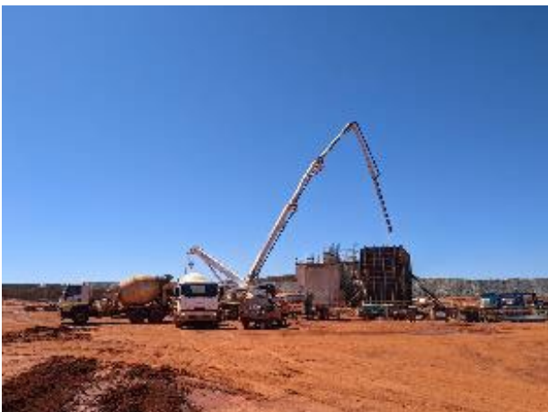
Figure 5: Pouring of the Fine Ore Bin foundations
