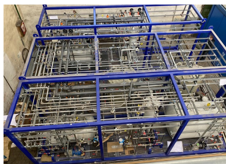
Optimisation plant under construction
