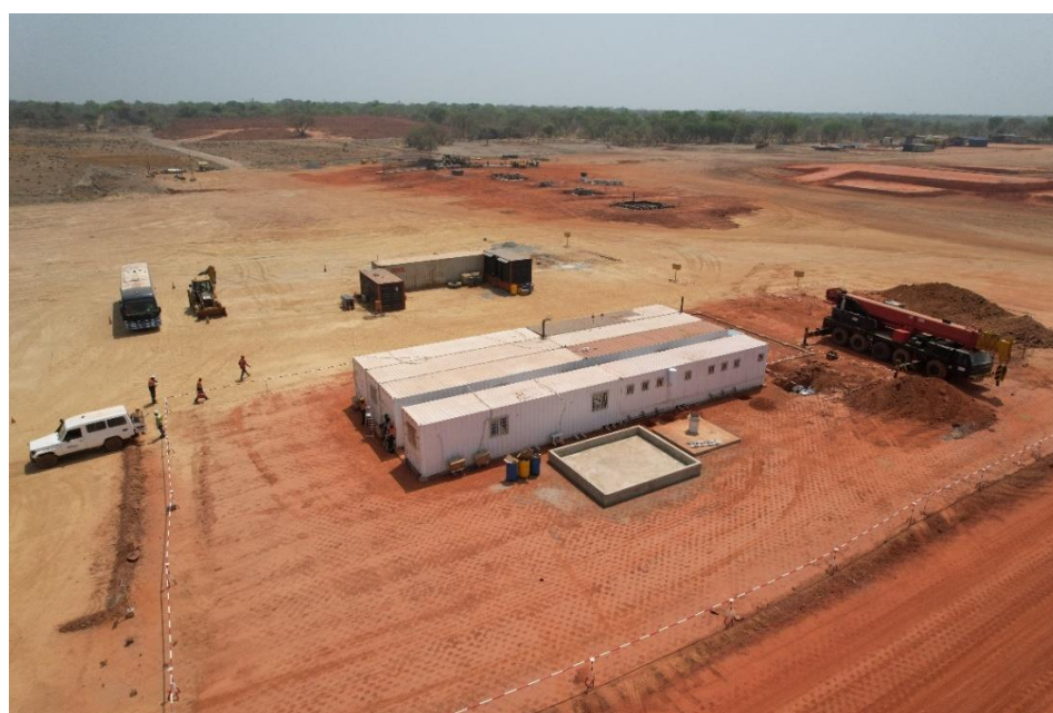
Image 4 -The temporary construction site offices at the Goulamina Project March 2023
