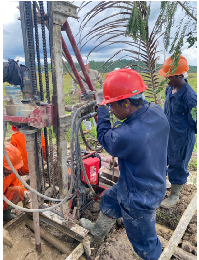
Drilling unit Onshore Kobi area
