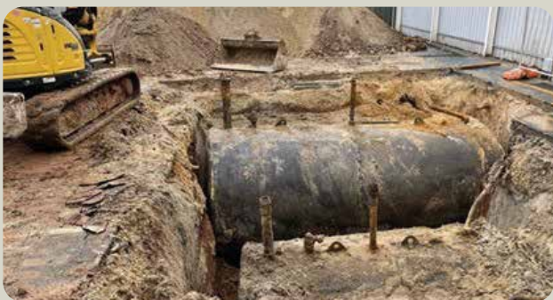
Underground Petroleum Storage System (UPSS) – One of the 37 UPSSs decommissioned, handed back or divested under our program of works to mitigate safety and environmental risks associated with UPSS.
