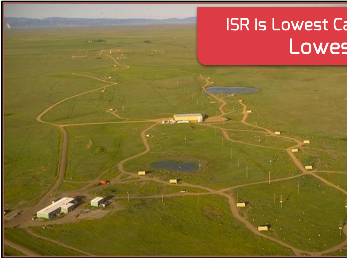
Cameco's Smith Ranch ISR Uranium Mine, Glenrock, WY
