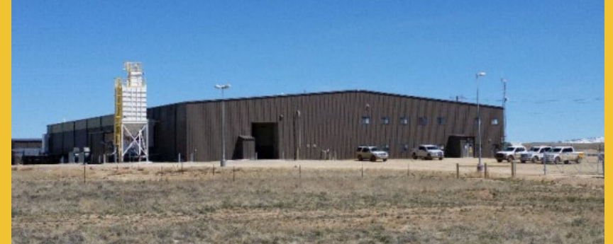
UR-ENERGY'S OPERATING LOST CREEK ISR PLANT
