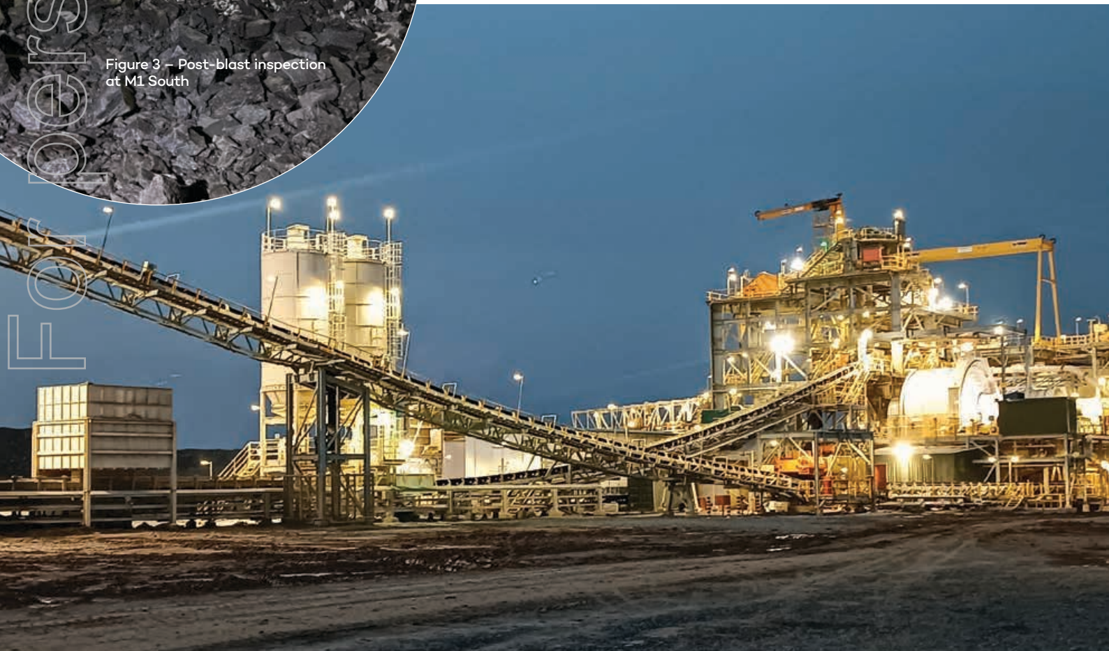
Figure 4 – Sanbrado process plant
