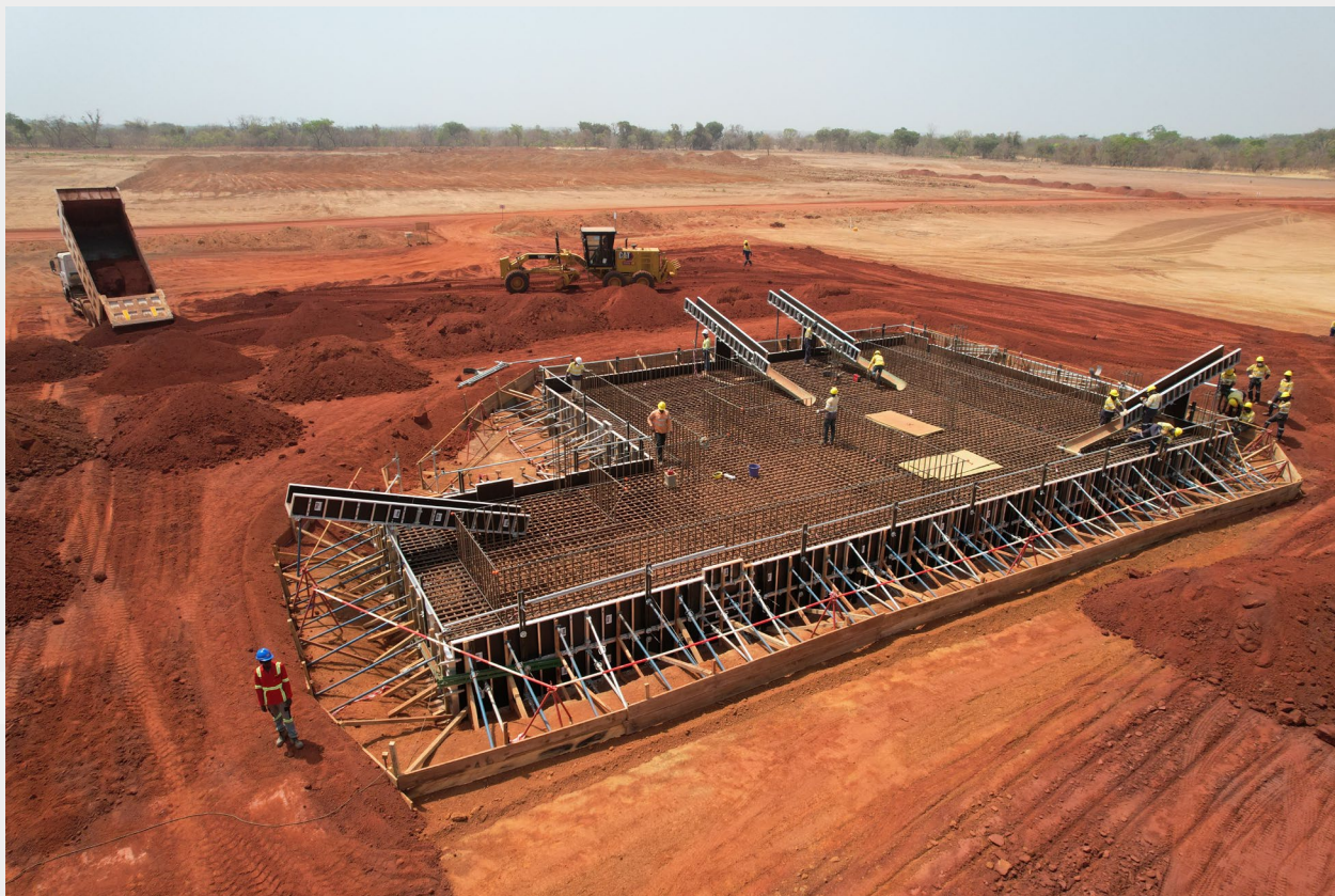
Ball mill raft slab preparations
