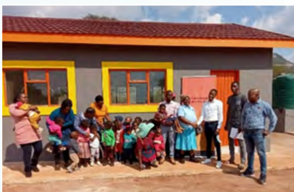
Minopex handed over a newly constructed creche in the Phalaborwa area, Limpopo, to the community.
