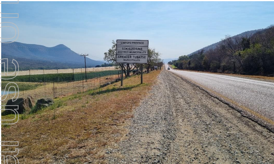
Paved Road to Site
