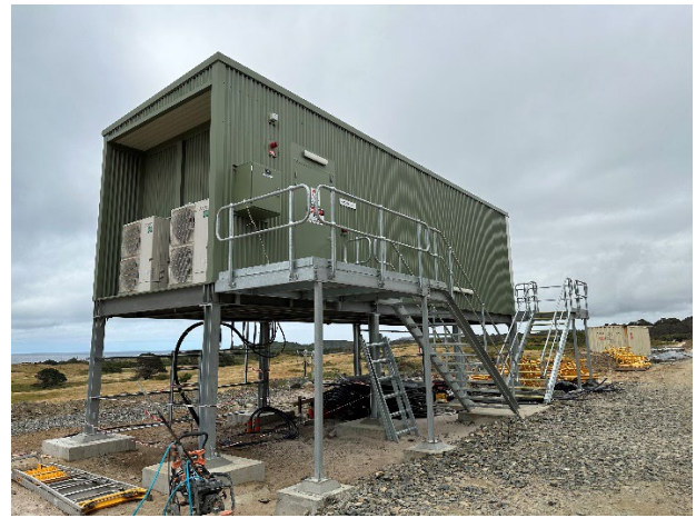
Figure 3 - Installation of MCC A & Electrical Termination
