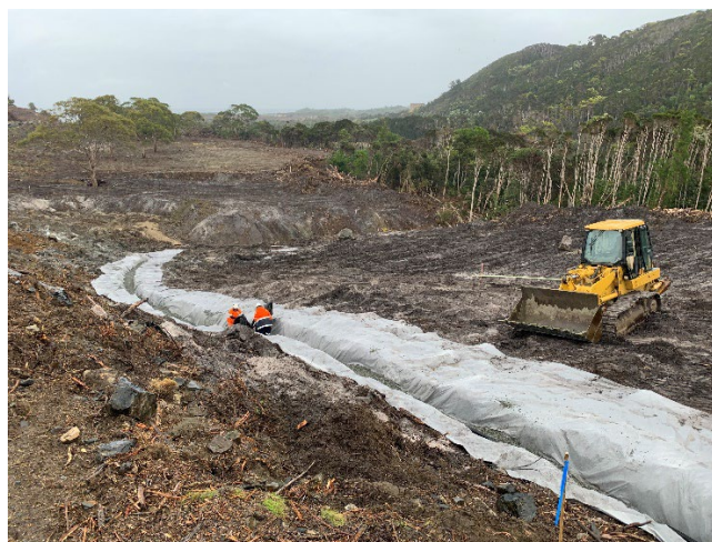
Figure 8 – Installation of Clean Water Diversion Drain
