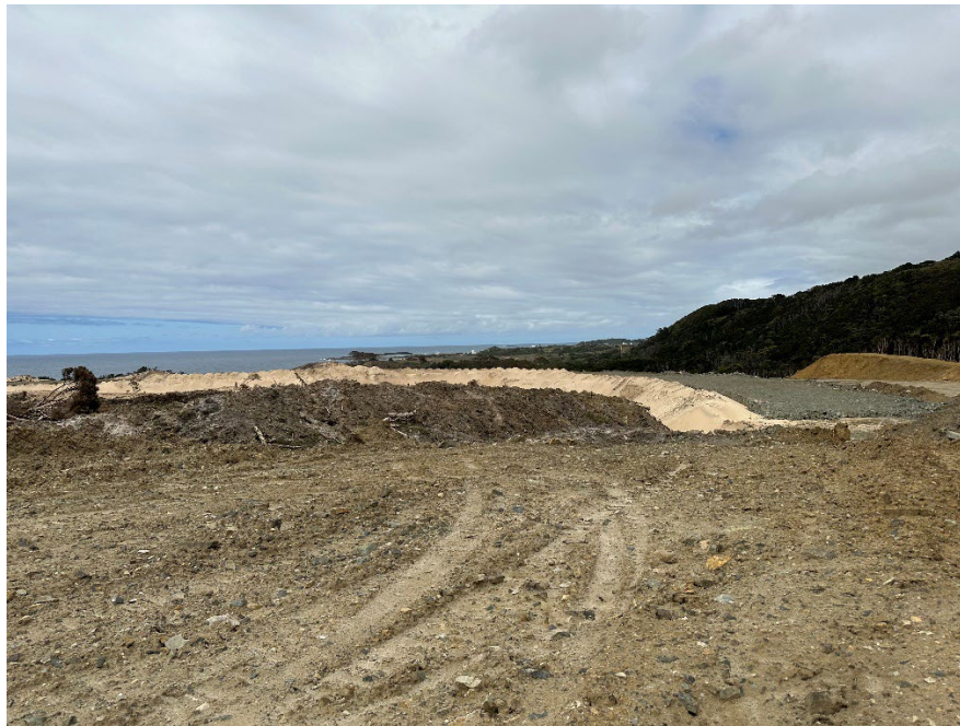
Figure 4 - Construction of South Western Wall of Tailings Storage Facility
