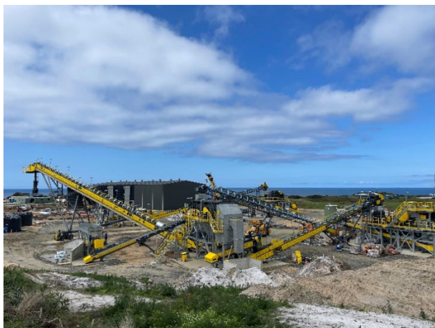
Figure 6 – Installation of Primary and Secondary Crushing Equipment
