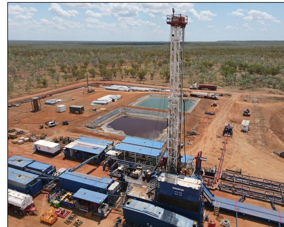
SLB 185 Rig drilling Carpentaria-3H in EP187
