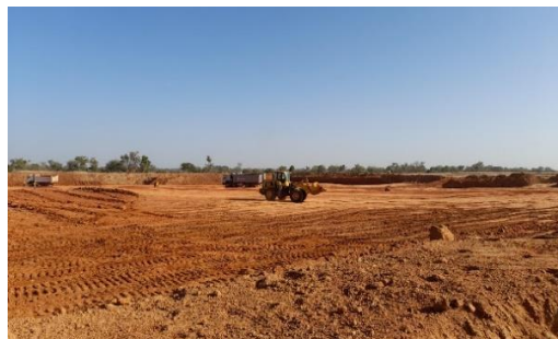
Mill clay excavation
