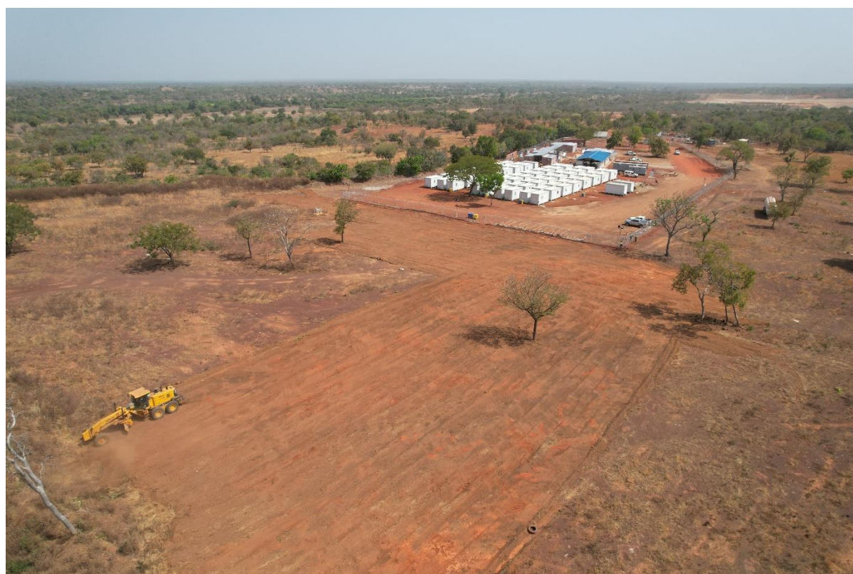
Clearing of permanent camp with temporary camp in background
