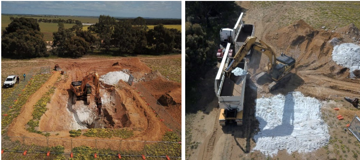
Figure 8: Test-pit in progress
