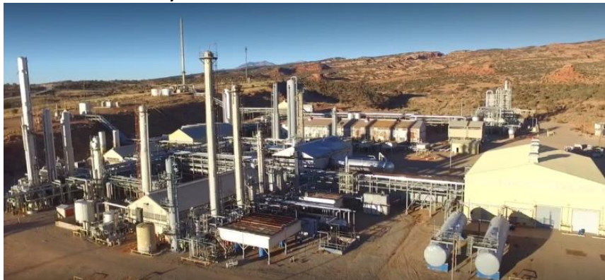
Paradox Resources “5 ½ Nines” Lisbon Valley Gas Processing Plant.
