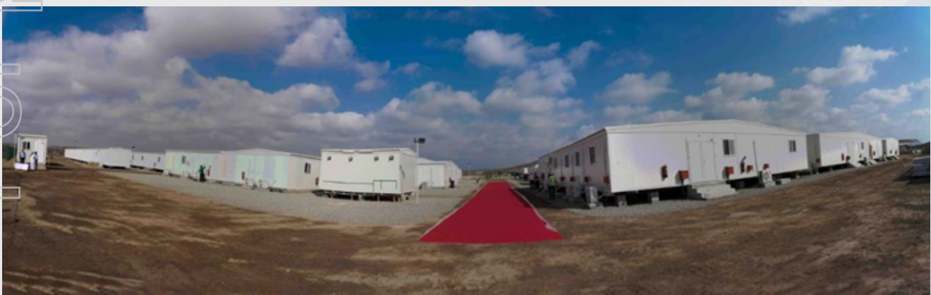
Accommodation village - wide angle
