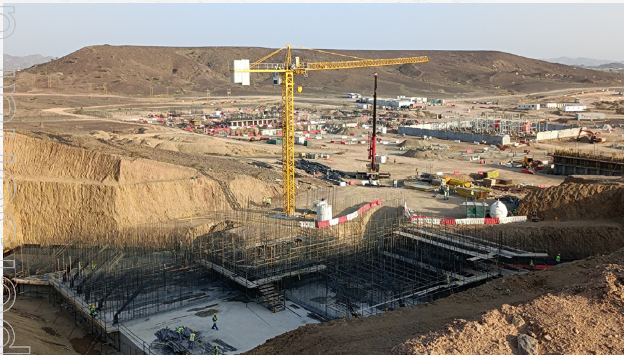
Copper-gold processing plant construction progress (late October 2022)
