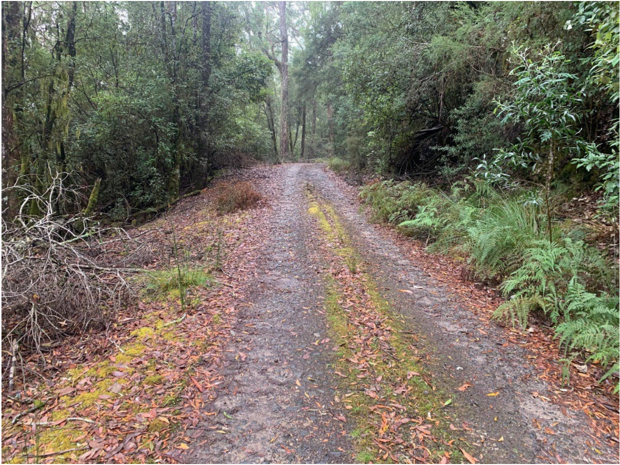
Image 2: Sheeted access road, established by forestry – Prospect Ridge
