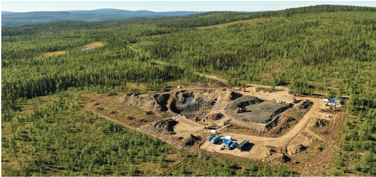
Figure 3 Talga's Vittangi Graphite Project trial mine 2022. Crushed ore is stored and processed offsite, and the open pit is being backfilled and rehabilitated to natural surface conditions. Environmental management includes 'smart' monitor bores with 24/7 live data transmission of groundwater conditions.
