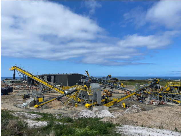
Figure 1 - Installation of Primary and Secondary Crushing Equipment
