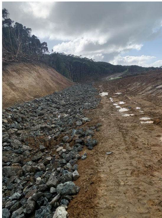
Figure 4 – Installation of Western Clean Water Diversion Drain for TSF
