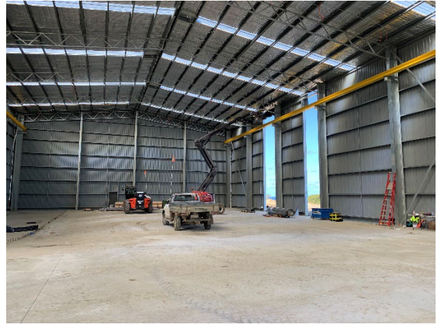
Figure 2 - Installation of Gantry Crane in Main Process Building
