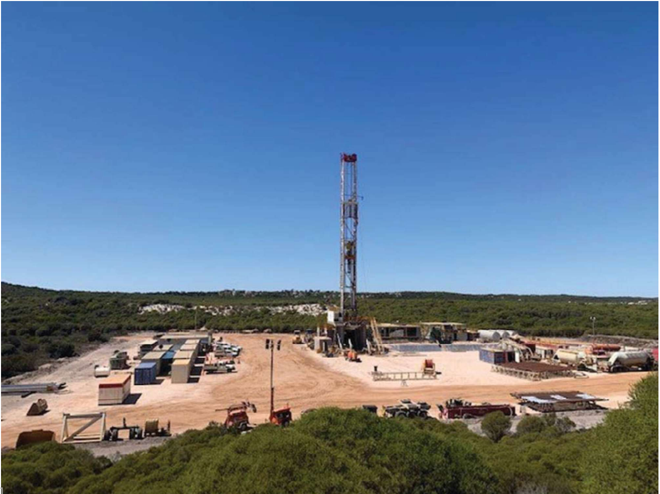
Figure 3: Ensign 970 drilling at Cervantes-1 location
