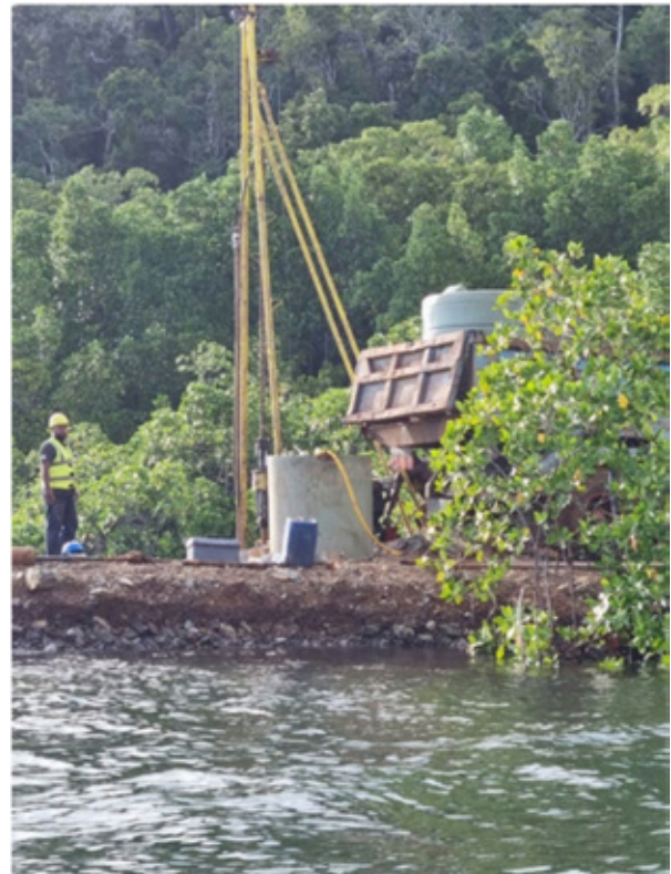
Figure 4 – Geotechnical Drilling for Wharf Construction
