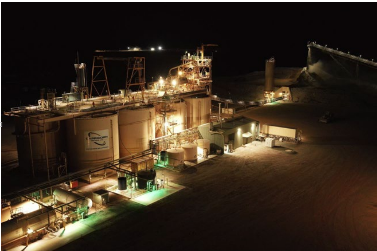
Processing plant at Karlawinda Gold Project
