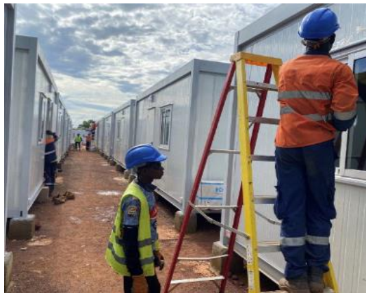
Installation of initial accommodation units
