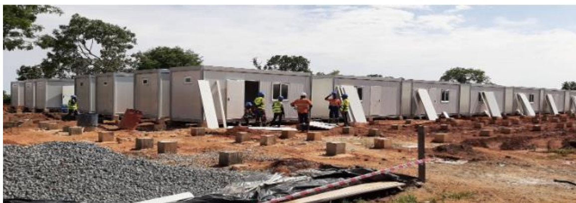
First 40 accommodation units and civil works for future units
