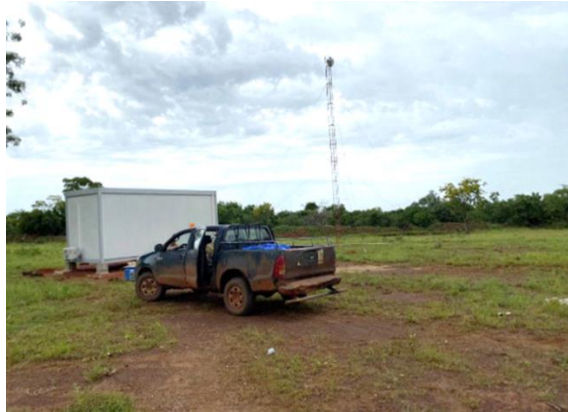
Site communications tower and control unit
