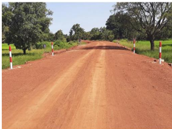
Completion of site access road
