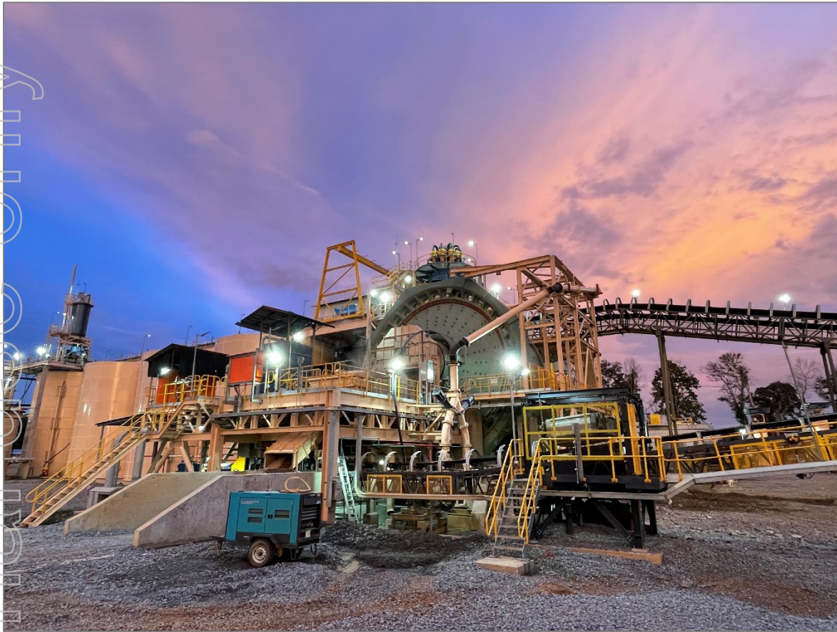
Figure 4 | Okvau Gold Mine processing plant
