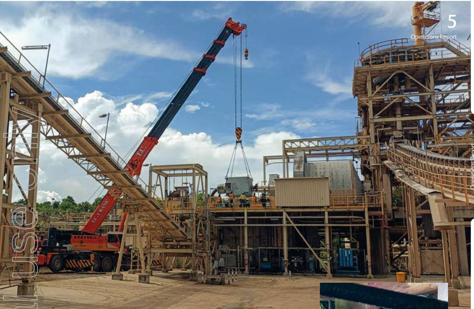
CR3 undertaking refurbishment works on Plant #2
