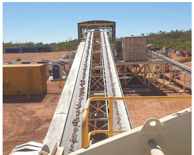
Ore Sorter at Browns Range Pilot Plant
