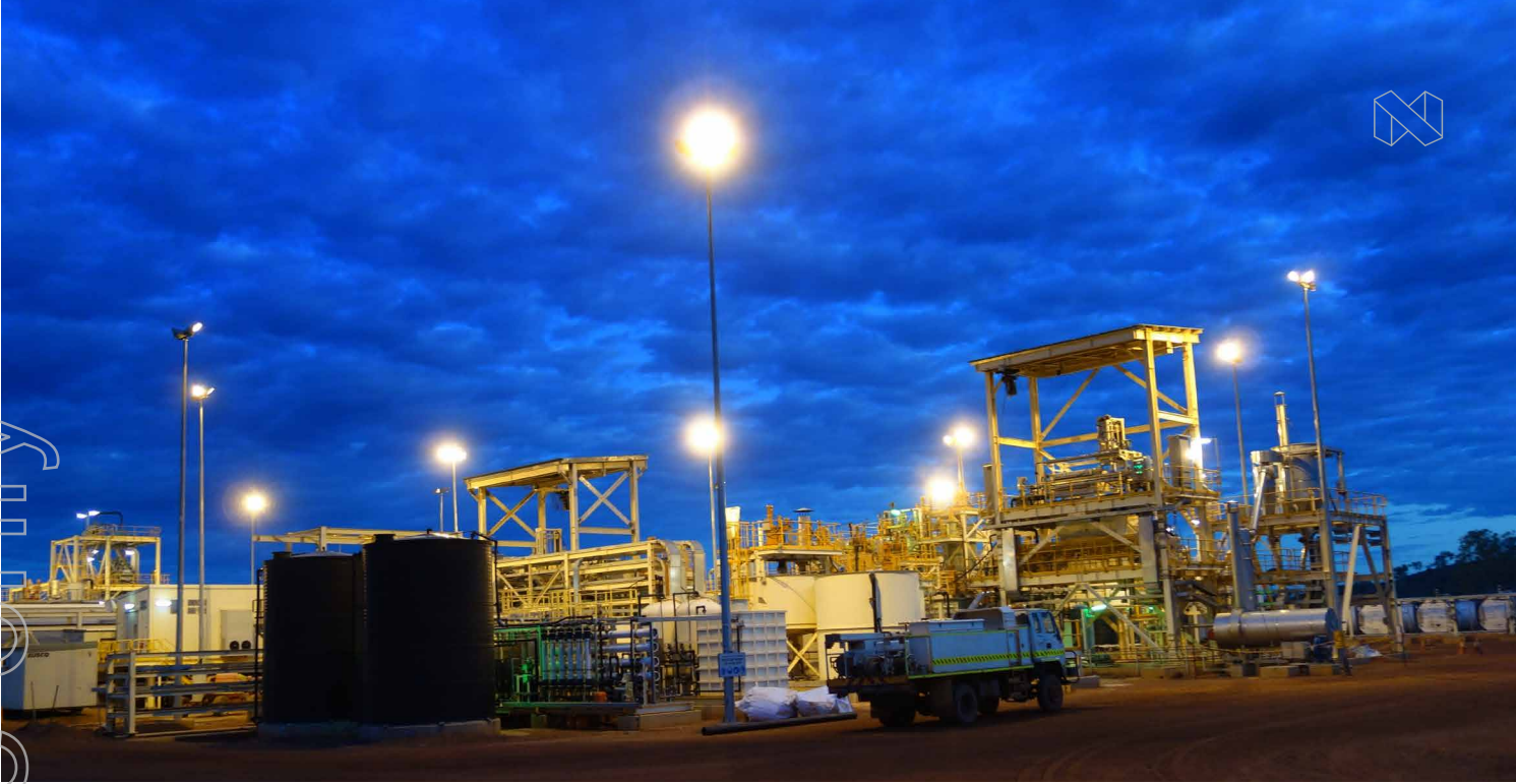
Browns Range Pilot Plant
