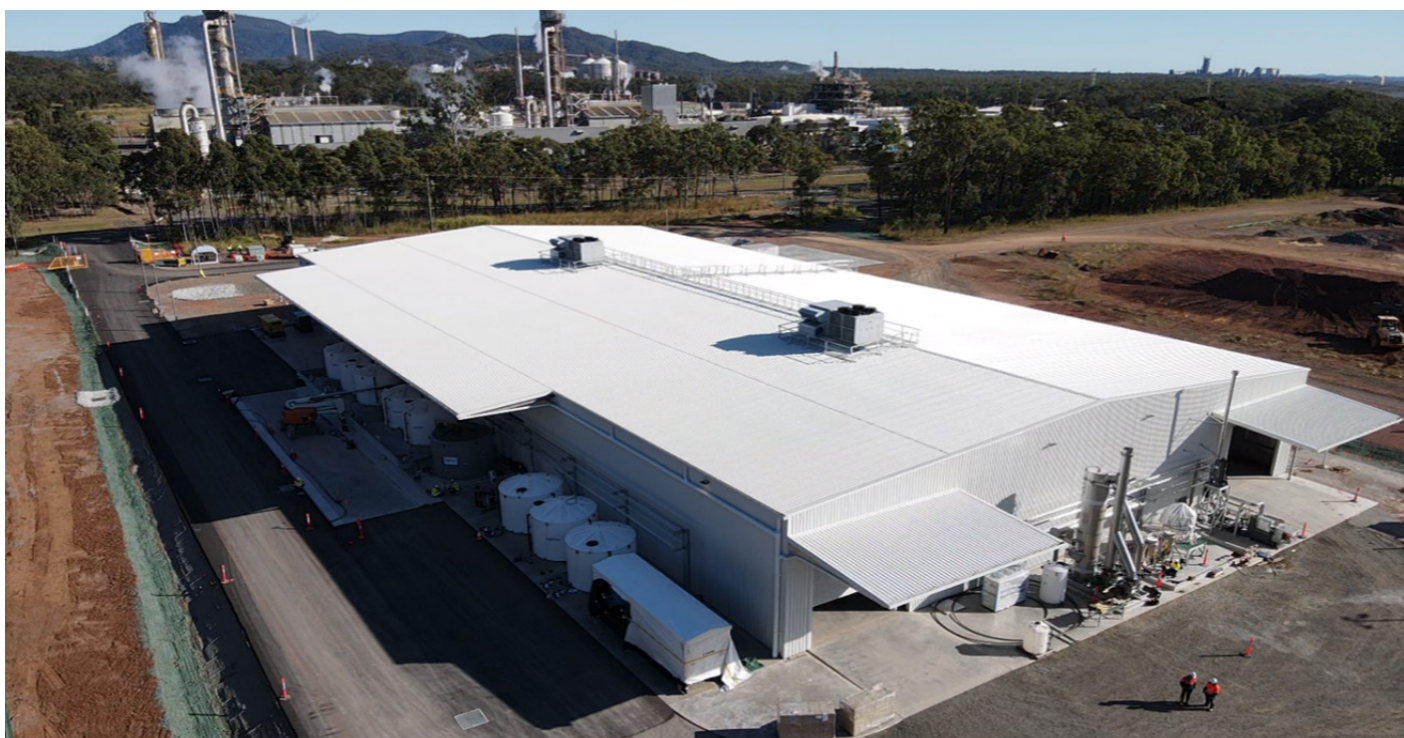
► Stage 1 PPF building at lockup stage
