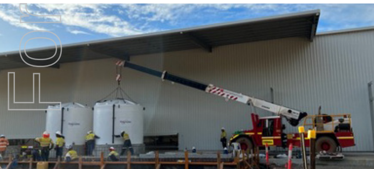
► Installation of PPF reagent tanks
