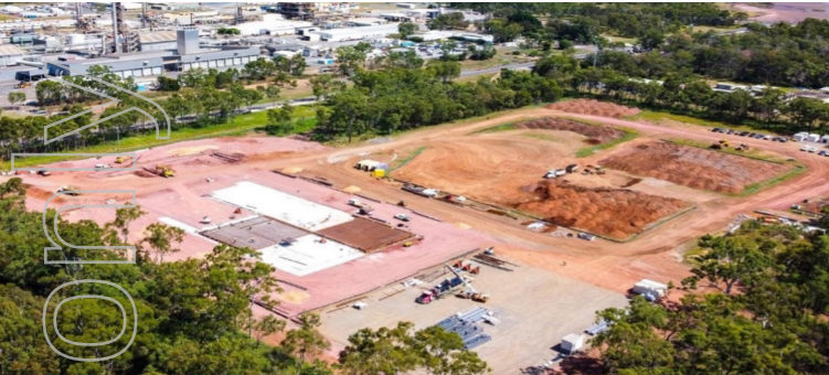
► Stage 1 PPF - preliminary earthworks
