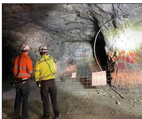
Underground development drive showing good ground conditions
