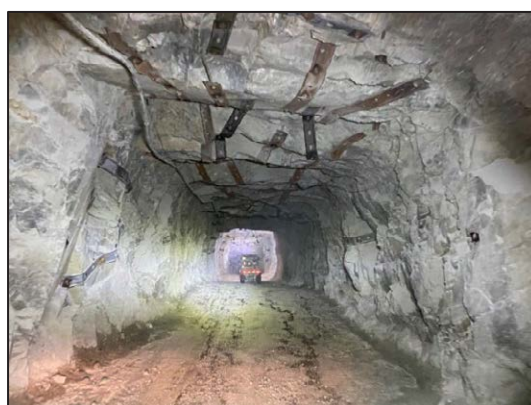
Underground intersection showing good ground conditions and existing services
