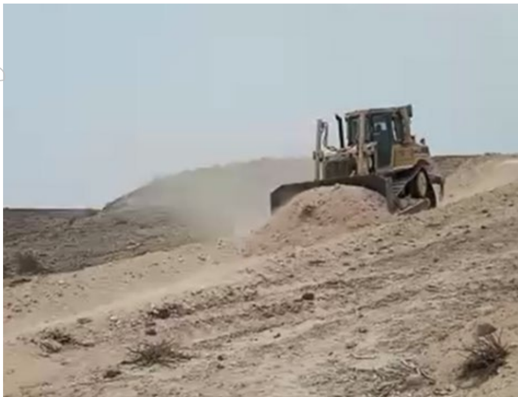
Figure 1: Dozer, operated by sub-contractor T-Angola, repairing a sandy section of access track.
