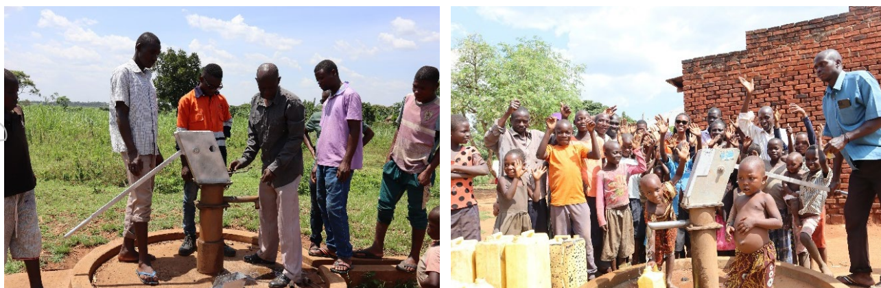
Figure 7: Serviced 11 community boreholes across the project area
