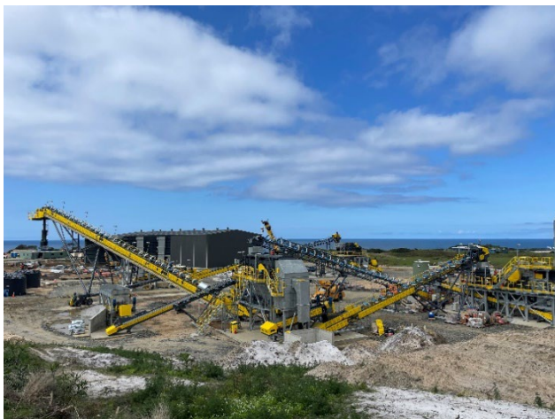
Figure 2 – Installation of Primary and Secondary Crushing Equipment
