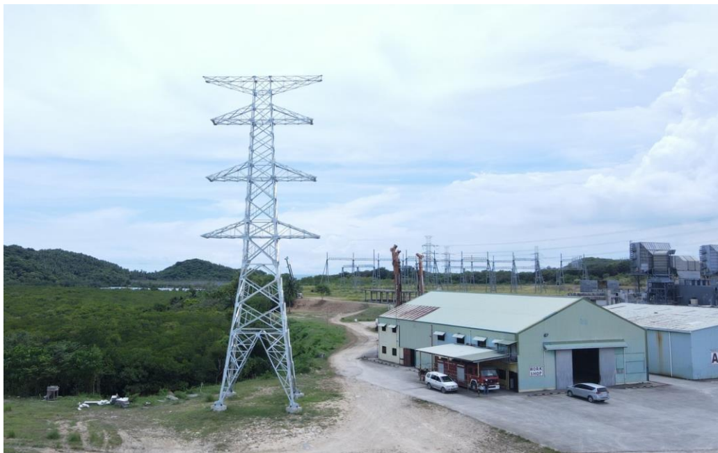
Transmission Towers for the EWC Transmission Line Under Construction
