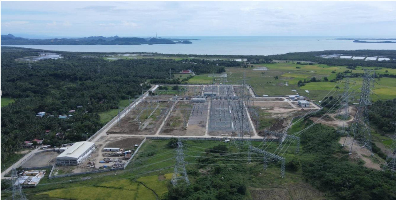
The NGCP New Pagbilao Substation Under Construction in Aug. 2022
