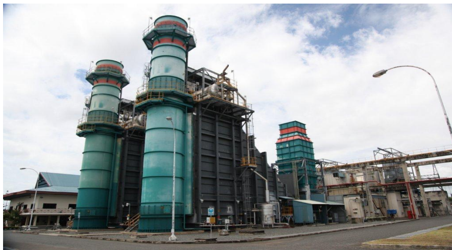
Sengkang Power Station in South Sulawesi, Indonesia
