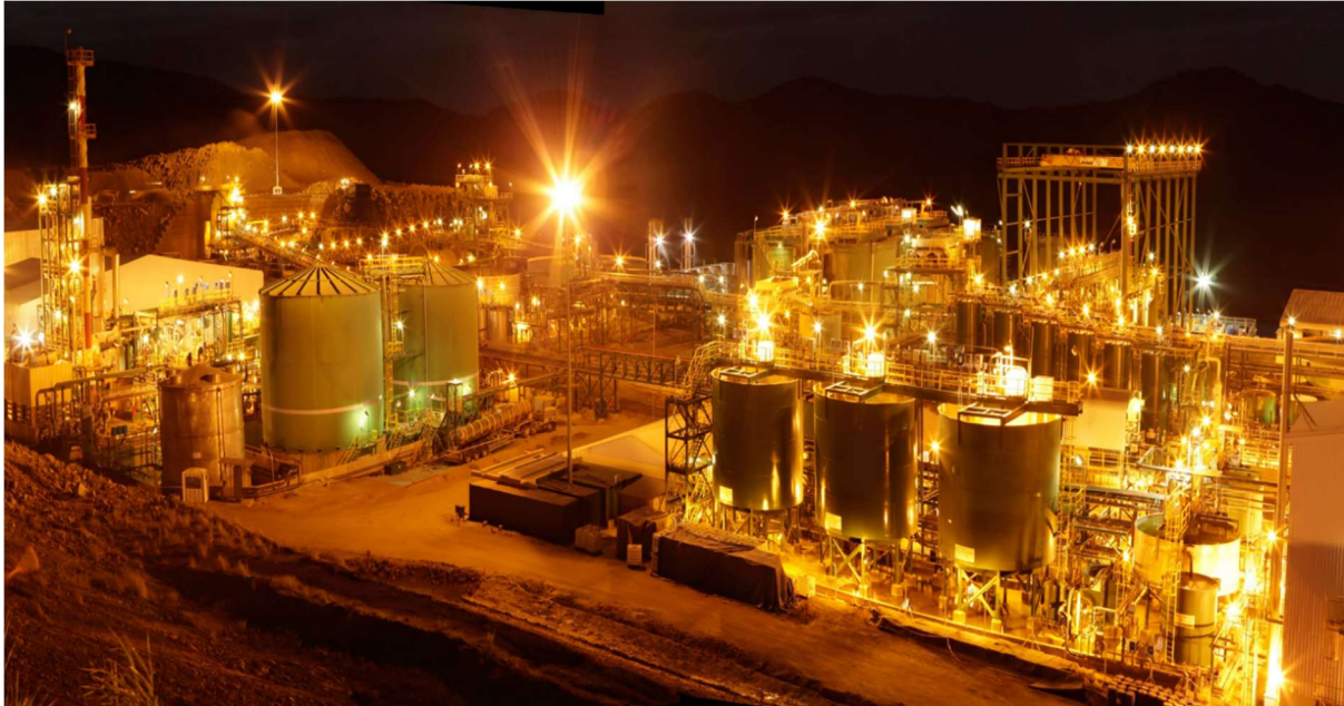
Image 2: Kayelekera Processing Facility
