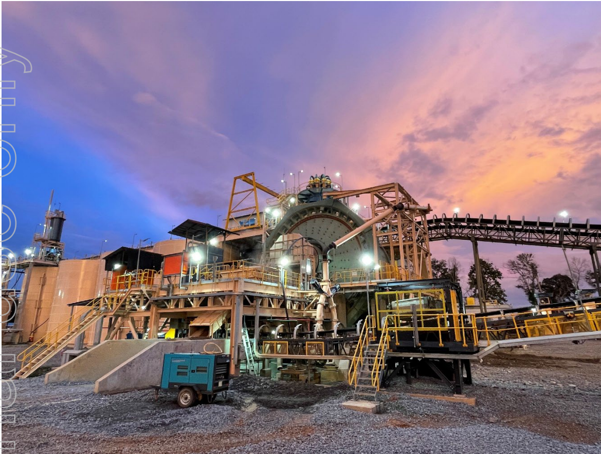
Figure 4 | Okvau Gold Mine processing plant
